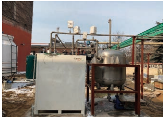
FIGURE 1. INSTALLATION OF SUNAMP UNIQ 80 PRODUCT WITH AN ORC SYSTEM IN SHIJIAZHUANG, CHINA
